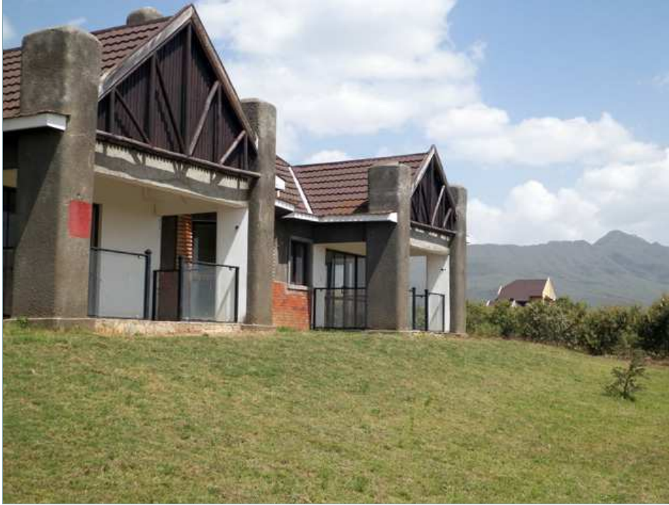
Houses under construction against a backdrop of Mt Longonot
