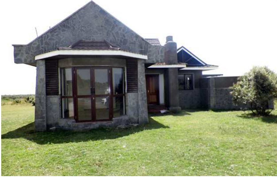
Ongoing landscaping at one of the houses
