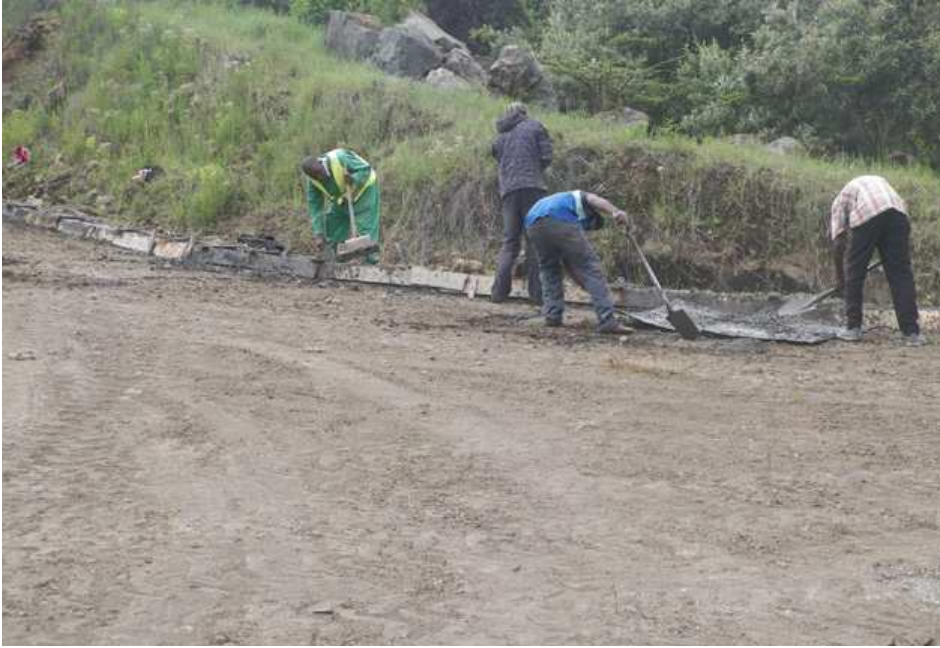
Roads construction masons concreting the beds for kerbing works
