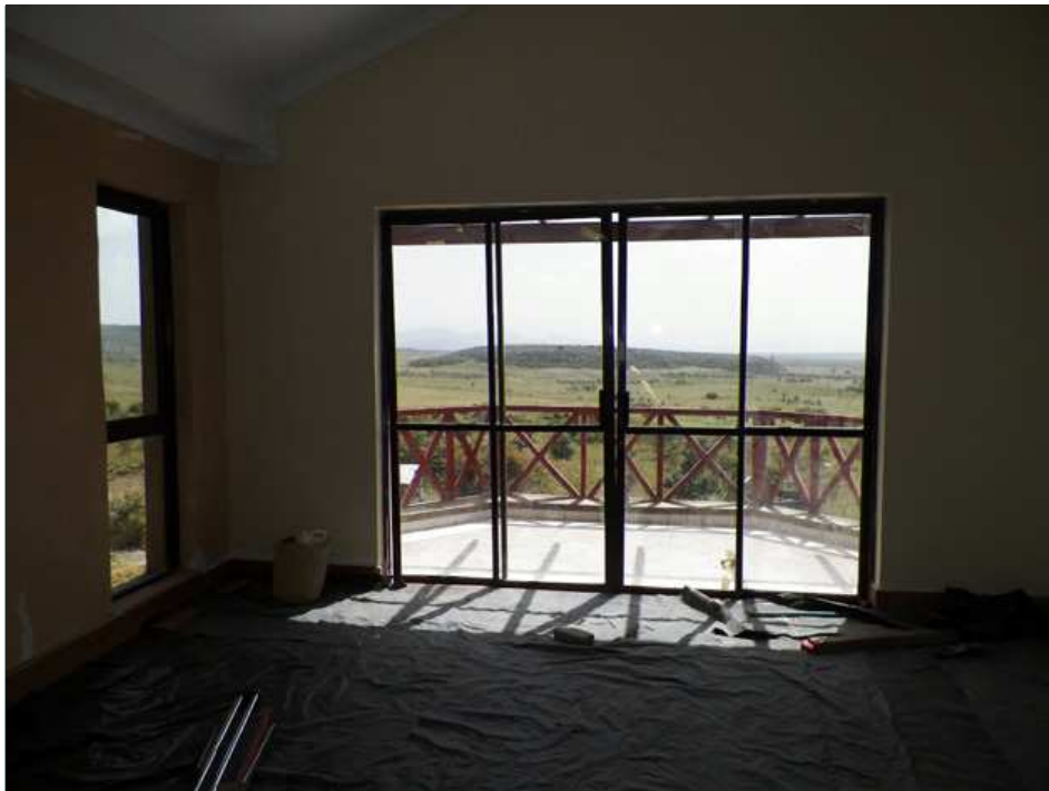
Inside one of the houses under construction
