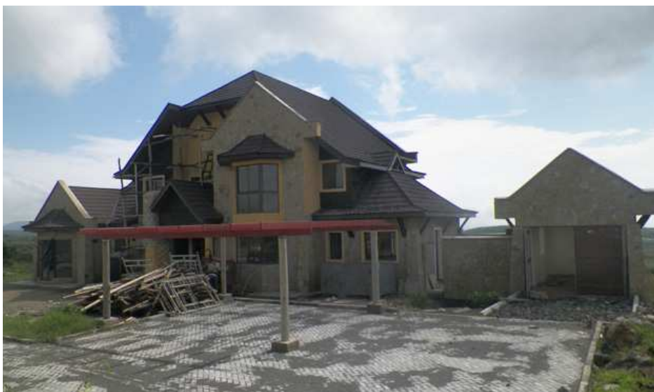
House Type C6 under construction
