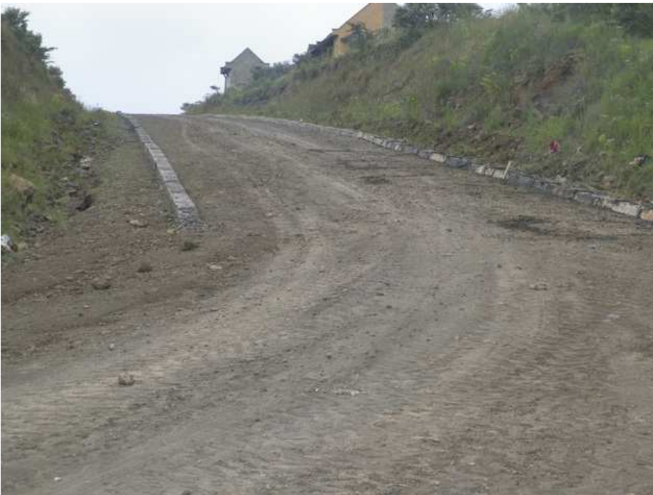
Laying kerbs on the spine road in Naivasha Gardens
