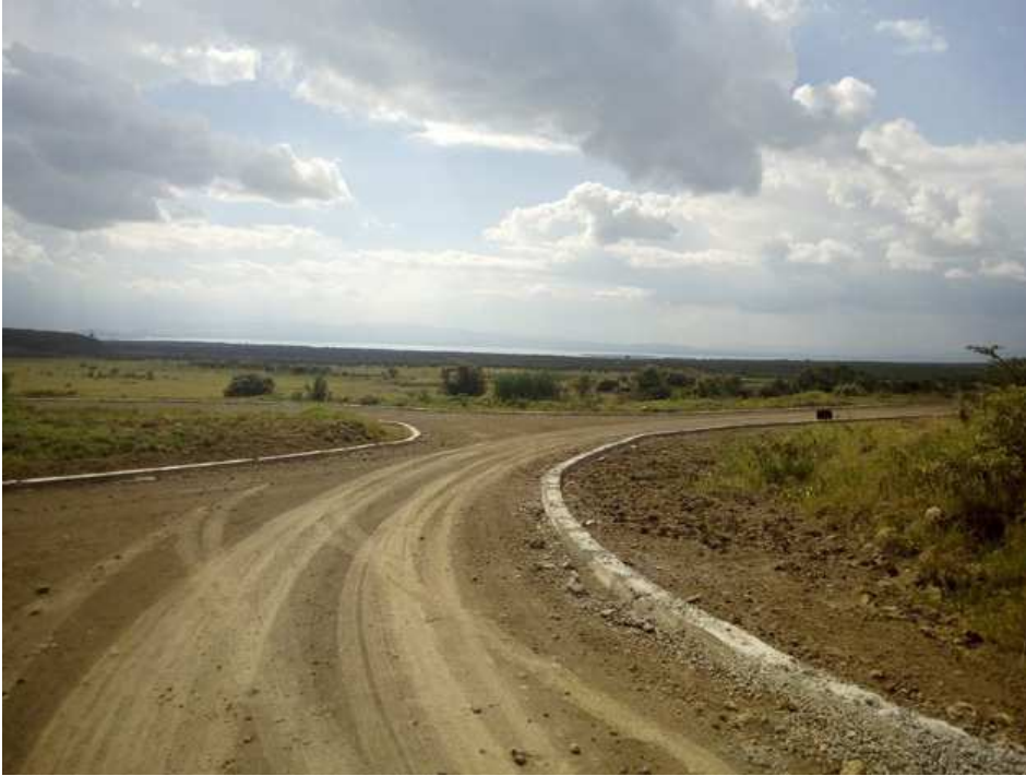
Laying kerbs on the main spine road
