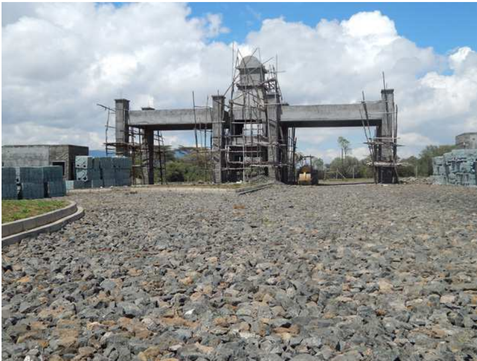
Mai Mahiu Gate under construction
